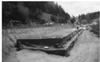
Installation of GeoSpec Lightweight fill Material
