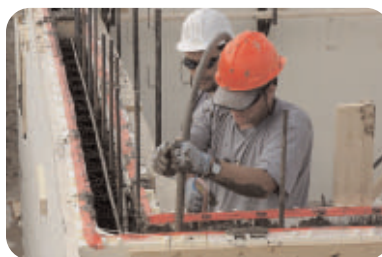
11 Vibrating concrete: in fast, out slow; straighten walls to string line
