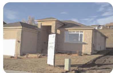
12 This is an Advantage Homes with a Difference project
