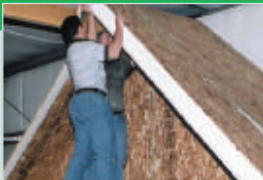
Use Insulspan SIP System for roof construction, ideal for vaulted or cathedral ceilings.
