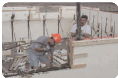
10 Placing concrete and vibrating: proper crew size required; 1" vibrator; clean site
