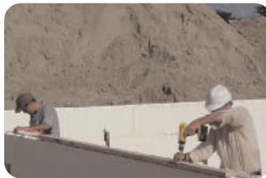
8 2 x 4 ribbon: attach around the top perimeter; set stringlines
