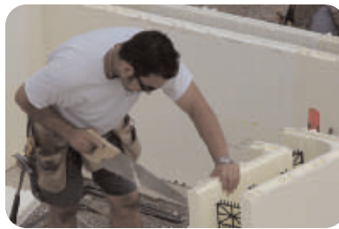
2 Stacking Advantage block: simple hand tools required
