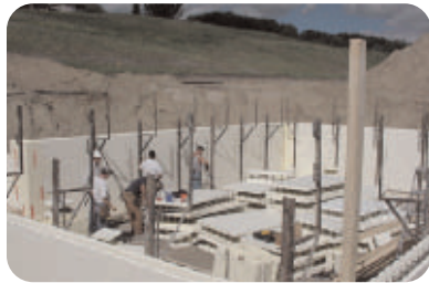
4 Install scaffold: at 3 rows high set scaffolding
