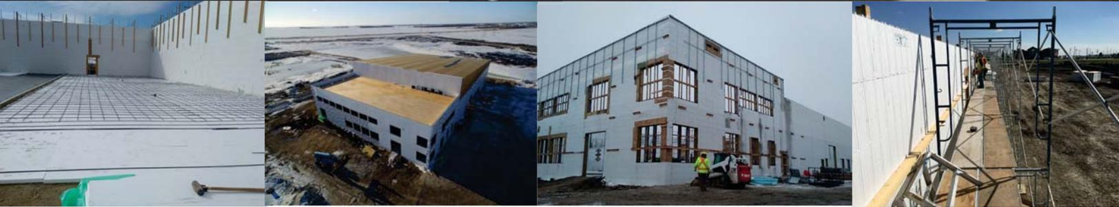
underslab for their cooler and freezer floors while providing the required higher compressive resistance for the entire 32,000 sq ft structure.
