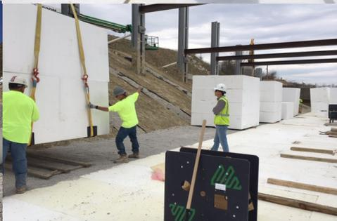
After a historic landslide damaged the runway of an airport in West Virginia, contractors turned to Plasti-Fab to supply 24,000 Cubic yards of geofoam for the repair project.
