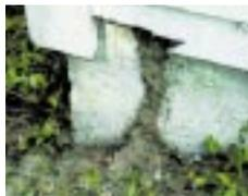
**PHOTO 1:** Subterranean termites build shelter tubes or mud tubes that serve as “climate controlled” access routes to a building. [Photo: Louisiana State University, Agricultural Center]
