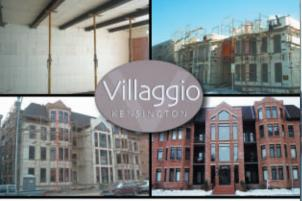
LaCosta Housing's Villaggio Kensington multi-family project. Features Plasti-Fab's Advantage ICF System for the exterior walls, interior partition walls and floors.
