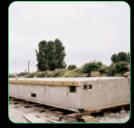
Concrete floating foundation with PlastiSpan flotation billets inside.
