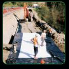
Construction crew backfills over the PlastiSpan lightweight fill blocks.
