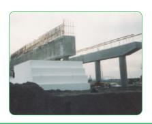
GeoSpec lightweight fill material can be used in road construction and landscape architecture applications where structural loading is an issue.
