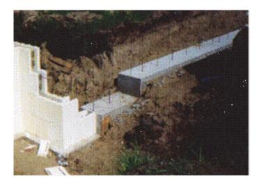
Figure 4: Photograph of Step Footings and Block
