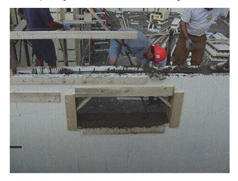
Figure 16: Photograph to illustrate RO Buck bracing.
