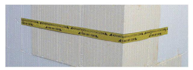
Figure 23: Photograph illustrating multi-strap on corner.
