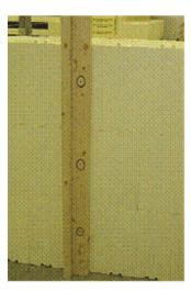
Figure 18: Photographs to illustrate placement of vertical scaffold braces.
