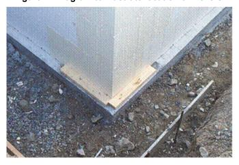
Figure 8: Photograph to illustrate placing of kickers.
