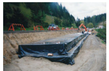
Figure 2 Installation of GeoSpec Lightweight fill Material
