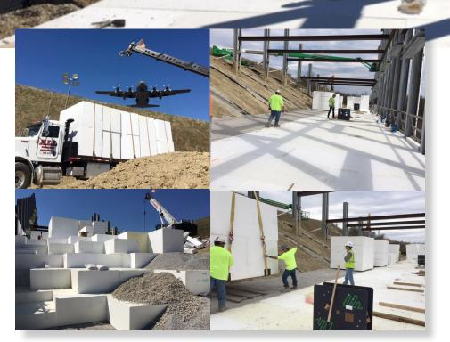
After a historic landslide damaged the runway of an airport in West Virginia, contractors turned to Plasti-Fab to supply 24,000 Cubic yards of geofoam for the repair project.
